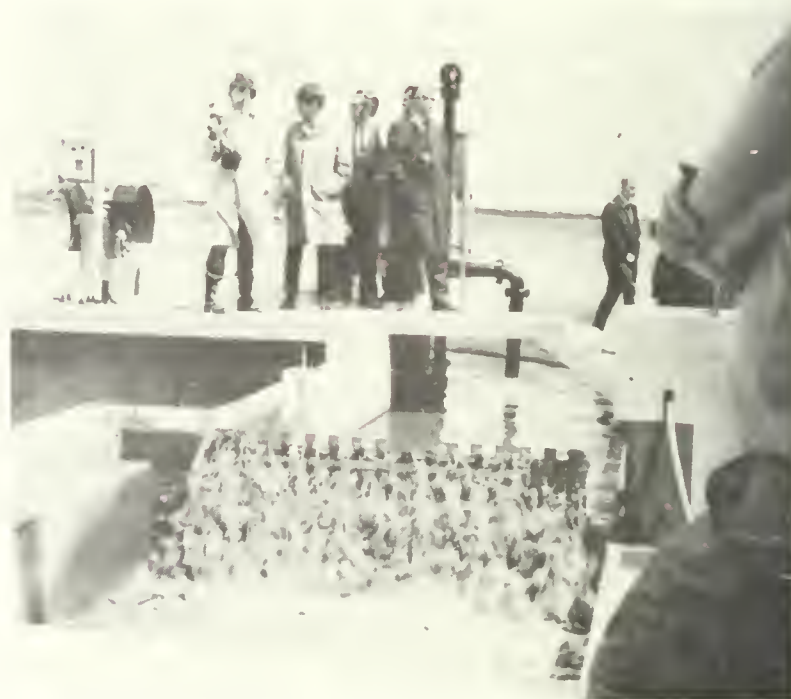
Figure 3.5.32 Brush-type aerator for oxidation ditch
